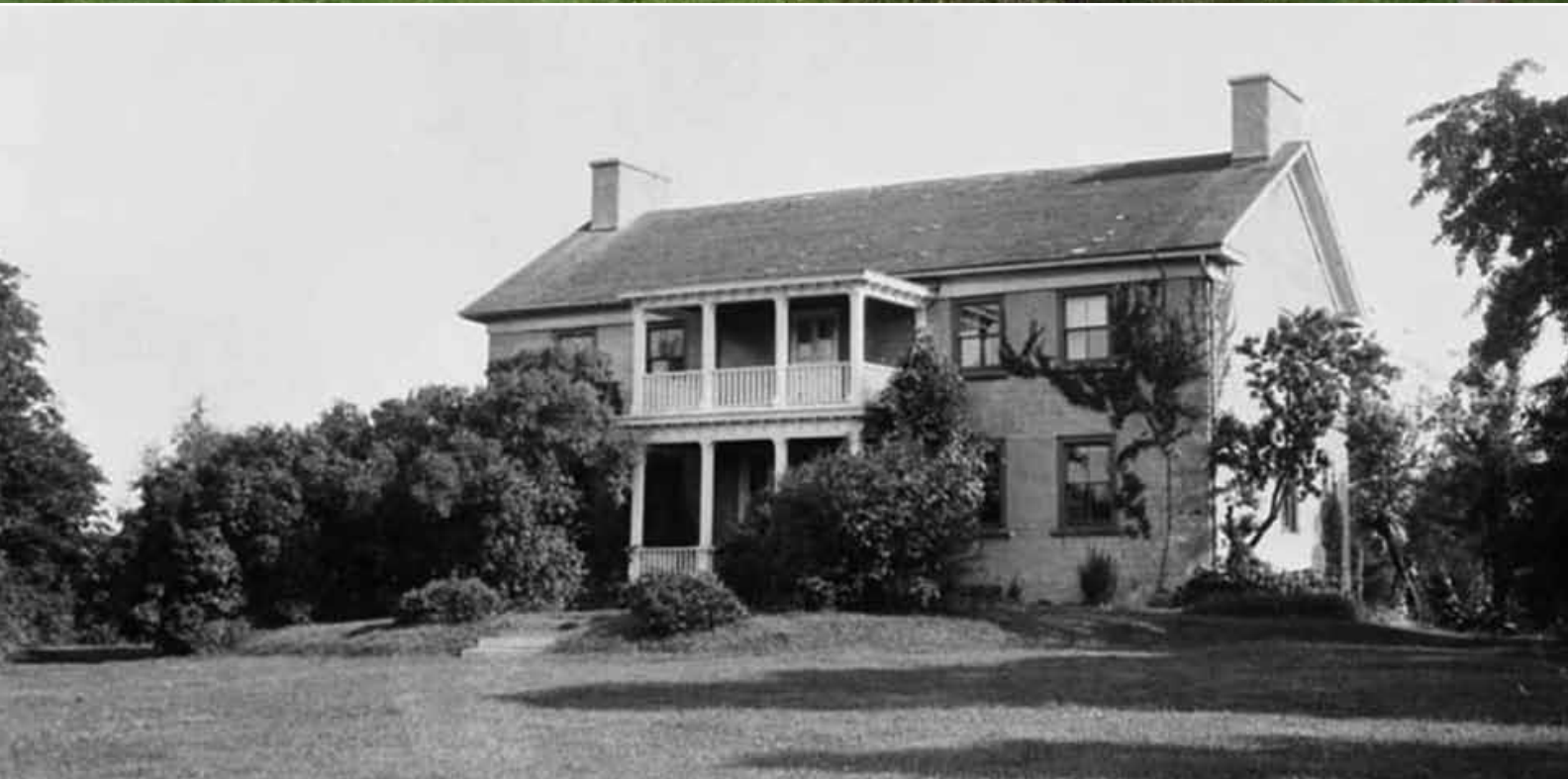
The DeCou house before it was destroyed by fire in 1950. PHOTO BY C. P. MEREDITH, COURTESY LIBRARY AND ARCHIVES CANADA.
